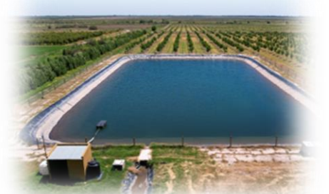
Recharge / Retention Ponds
